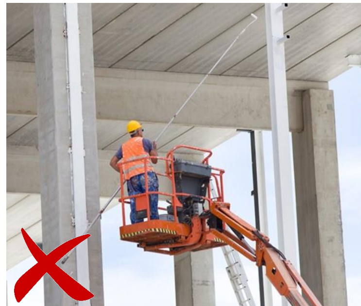
No body harness or restraining belt being used.
