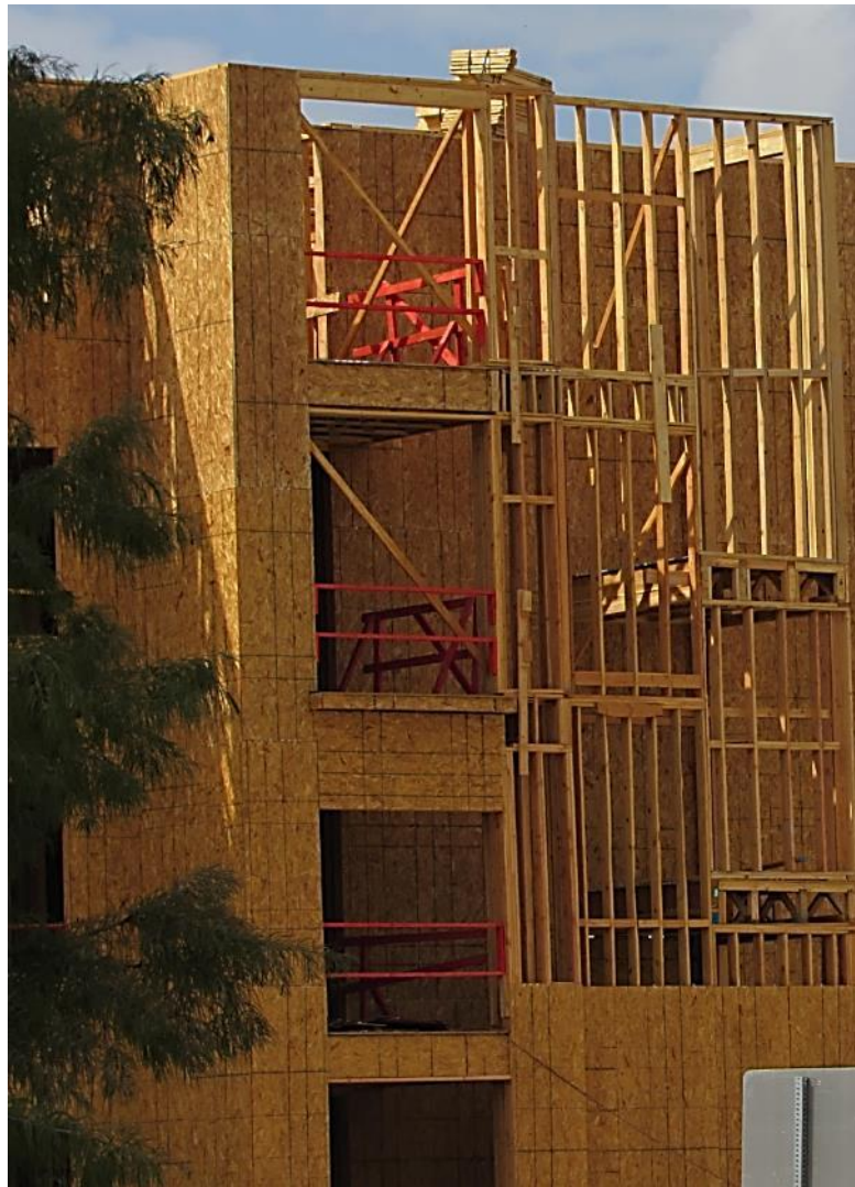
Guardrails installed and maintained.
