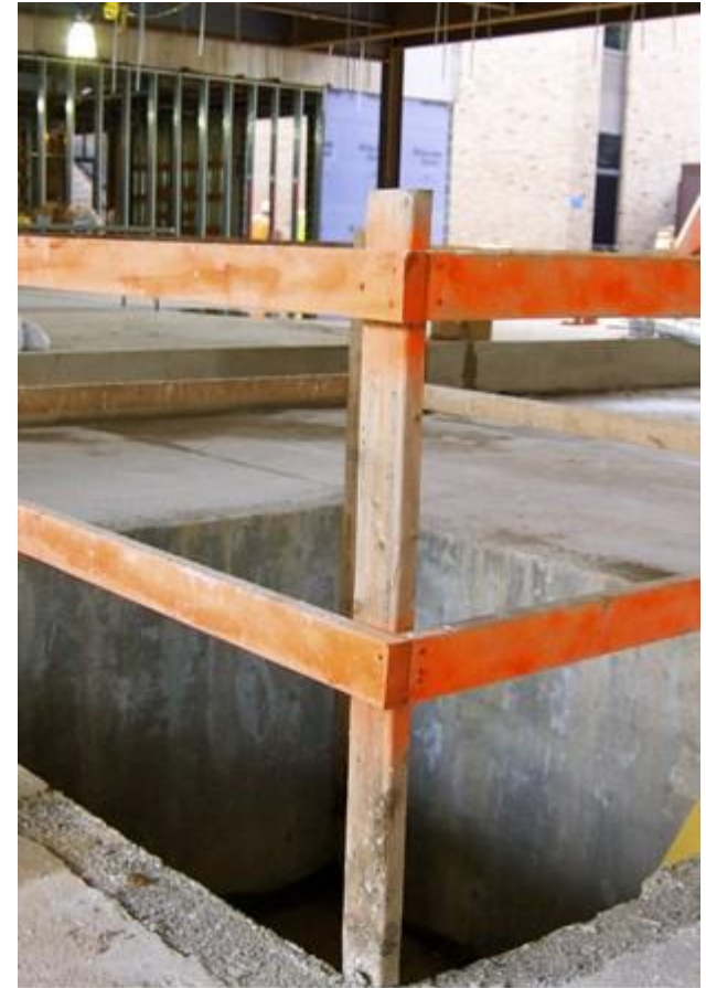
Image: J. Vinton Schafer & Sons, Inc. and CCBC Catonsville/eLCOSH.org
