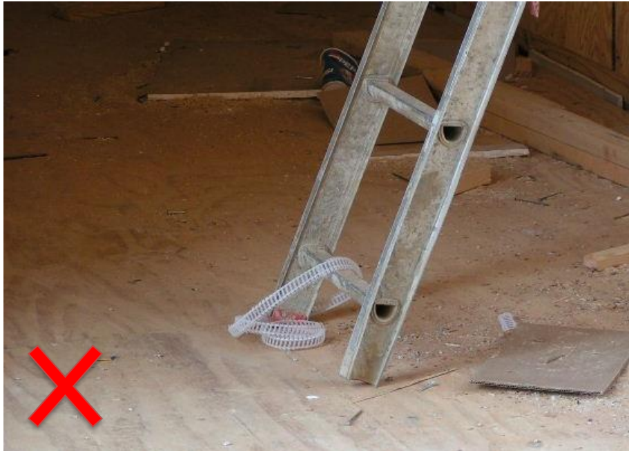
Extension ladder missing foot assembly and foot pads. This appears to be the top portion of an extension ladder that has been taken apart.
