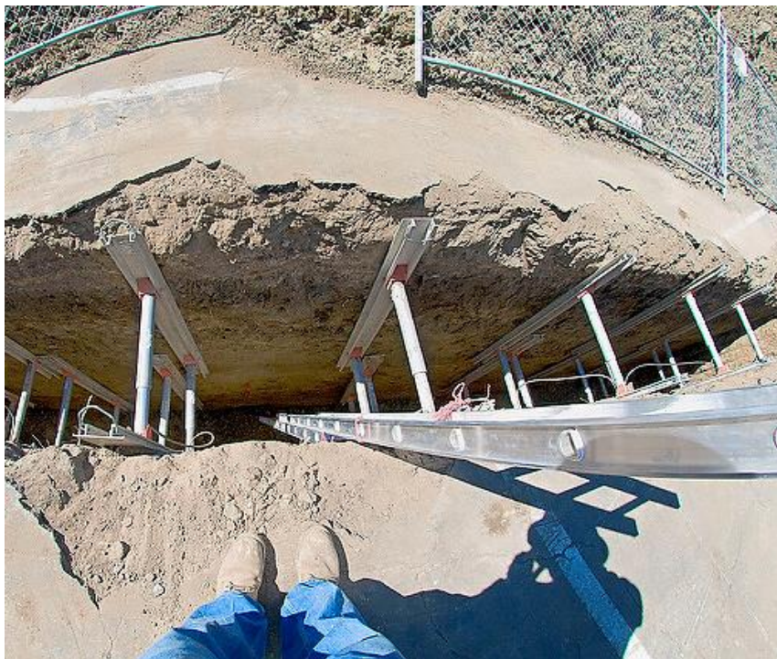
Example of standing above a system of hydraulic shores. (*4)
