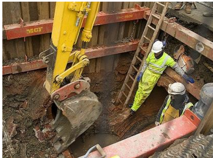
Example of workers inside of a timber shoring system. (*5)
